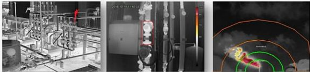
Fire detection, hot-spot and flare monitoring
