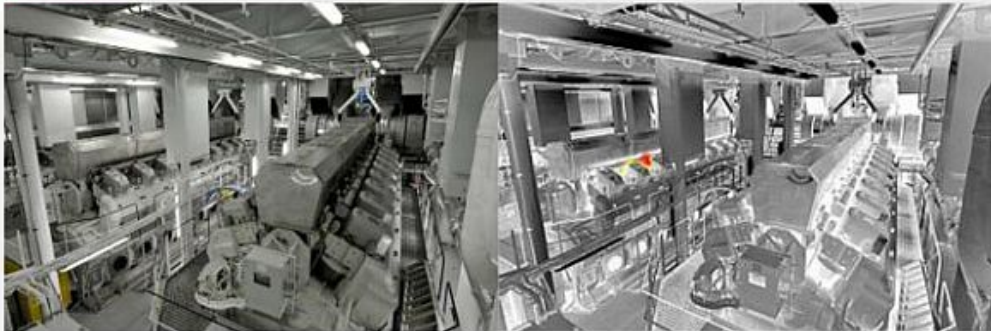
FlameGuard: Fire detection in a machine room
