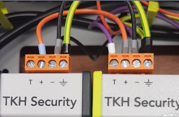
Tamper switches are connected to the Pluto network controller. The purple cable (T) on the Pluto network controller is de tamper input.
