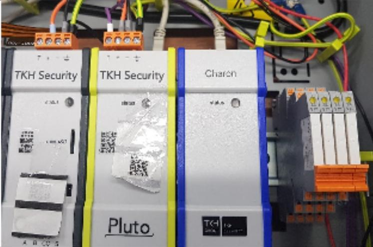
We advise you to leave some space on the left side for a possible expansion of the Orion door controllers and to place any necessary relays on the right side.
